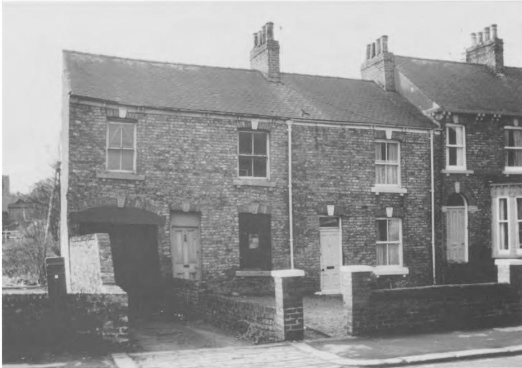
**Fig. 7.** Subsidence-damaged houses on Princess Road, Ripon [SE 3156 7266] showing a sagging mode of failure. These properties have suffered differential subsidence caused by settlement of peat within a large amalgamated subsidence hollow; active gypsum dissolution may also have contributed to the problem. This property has recently been demolished and has been rebuilt in a similar style on a piled foundation.
