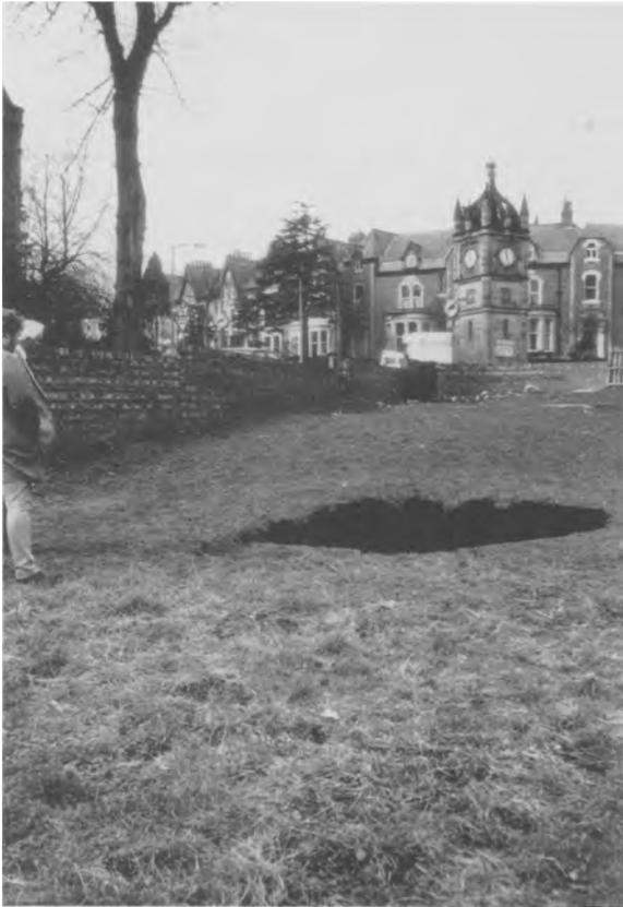
**Fig. 10.** Subsidence hollow that appeared in March 1987 near the Clock Tower [SE 3132 7281] in Ripon. This subsidence feature (5 m long, 3.2 m wide and 2.2 m deep) is in an area of glacial till adjacent to a large area of amalgamated peat-filled subsidence hollows (extending along Princess Road; see Fig. 7).
