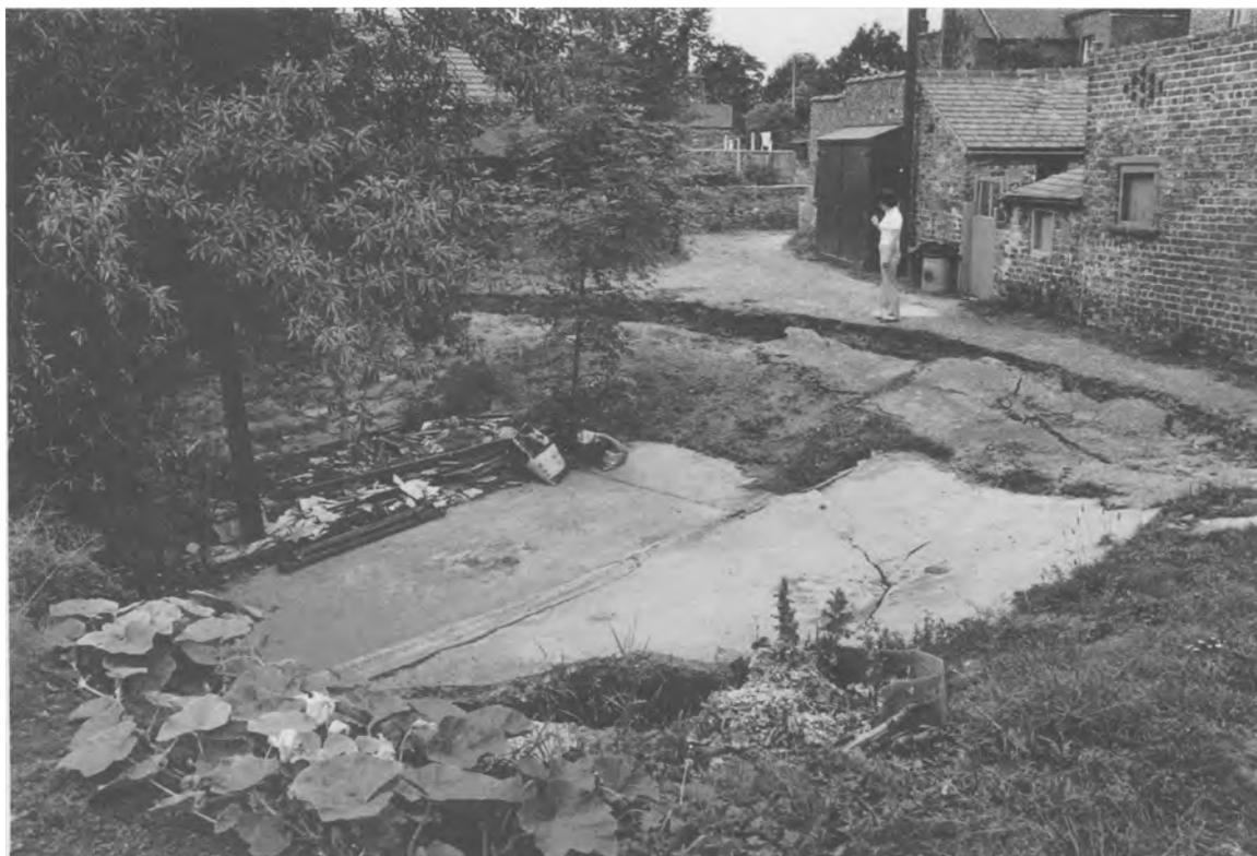
**Fig. 6.** Subsidence hollow that formed on 28 July 1979 behind houses on Magdalens Road, Ripon [SE 3170 7192]. This hole was filled in and subsided a similar amount in 1980. (Photo: Acrill Newspapers)
