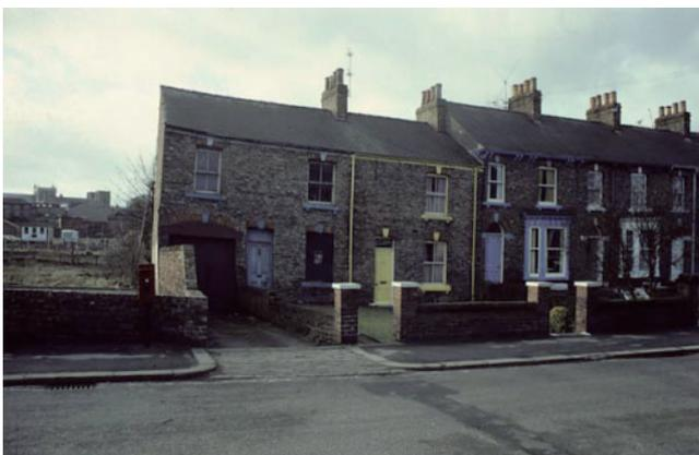
**Fig. 3.** Sagging building damage category 5 caused by gypsum dissolution and associated settlement on peat deposits, Princess Road, Ripon (Cooper 1998).
