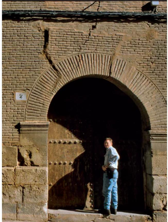
**Fig. 4.** Category 5 damage to a historic building in Calatayud, Spain (note the concentration of the damage in the arch). This is a hogging mode of failure with loss of support to the right of the picture.
