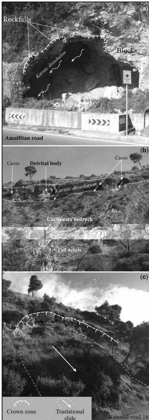
**Fig. 13.** Karstic dissolution and landslides along a detrital slope: (a) rock falls on the 'Amalfitana' road; (b) caves in instable conditions along the contact between inclined detrital body and limestone bedrock; and (c) translational slide on the National Road 18.
